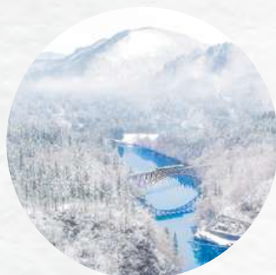
Daiichi Tadami River Bridge and Tadami Line / Fukushima
